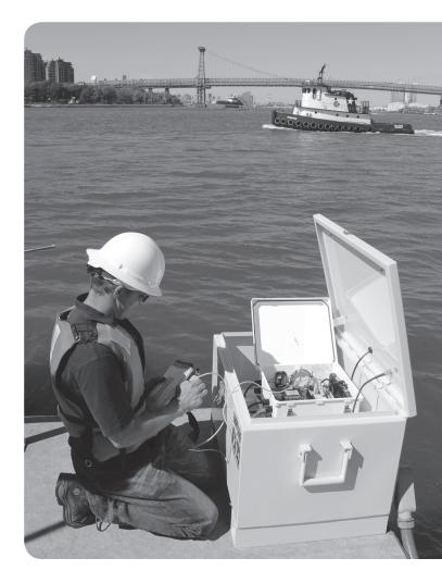
An example of a NEMA enclosure where the DCP Signal Output Adapter is wired.
